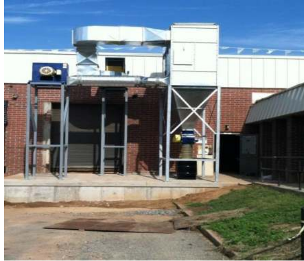
40 HP Drum Storage
