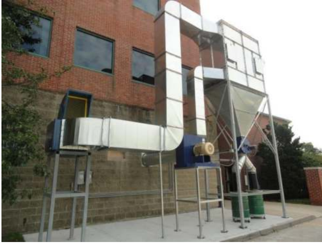
30 HP Drum Storage
